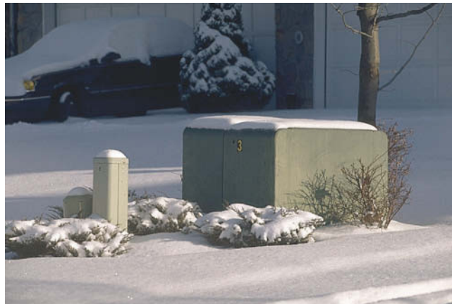
FIGURE 38-7 A pad-mounted transformer, if damaged, poses a serious threat.
